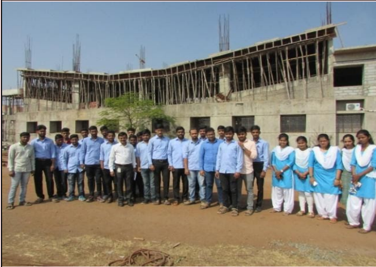
Field Visit to "FORMWORK" at Ashokrao Mane Medical College, Vathar. (15/01/2020)
