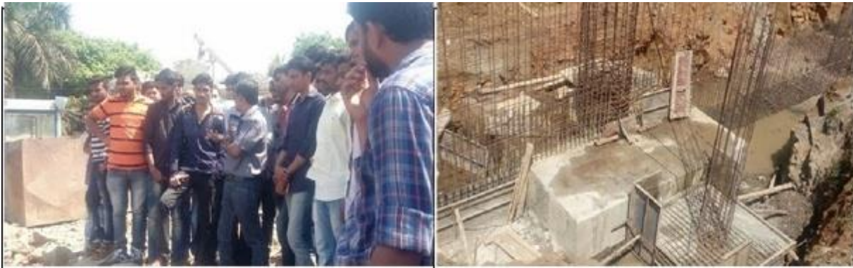
Industrial Visit to Foundation Site
